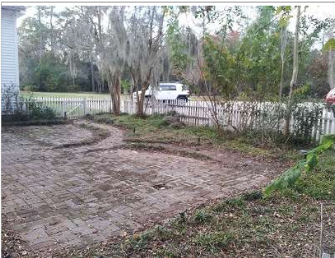
Clean up and re-set bricks in patio area.
