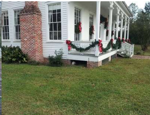
Repair green lattice and paint around base of Richmond House
